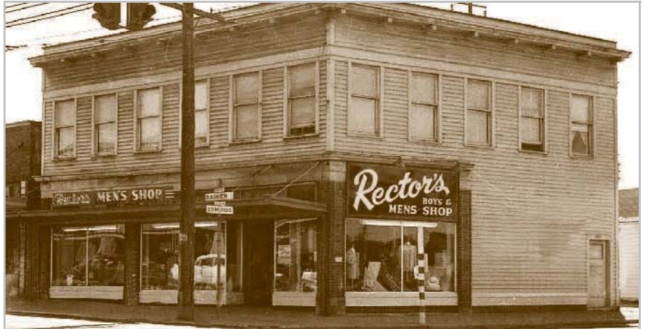
The building that would become Rector's was constructed in the spring of 1912 at a cost of $4,000. Photo: RVHS.
